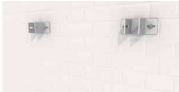
1st. Double "T" SCH-1-59 fixings.
