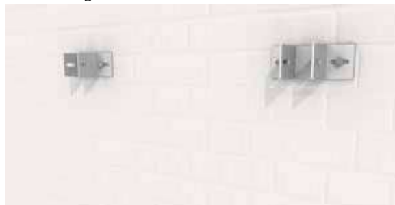
1st. Fixings with double “T” SCH-1-59
