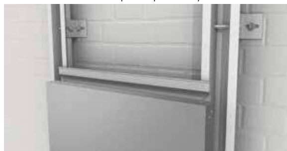
4th. STACBOND® composite panel tray
